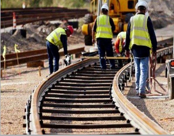
RE CONSTRUCTION OF SİNCAN- ANKARA-KAYAŞ TCDD RAILWAY LINE (BAŞKENTRAY) PROJECTS
