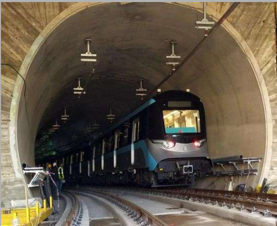
DUDULLU-BOSTANCI METRO PROJECTS RAILWAY SUPERSTRUCTURE WORKS
