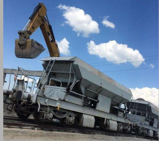
ANKARA MALIKOY BAŞKENT ORGANIZE SANAYİ BÖLGESİ CONNECTION LINE CONSTRUCTION WORKS
