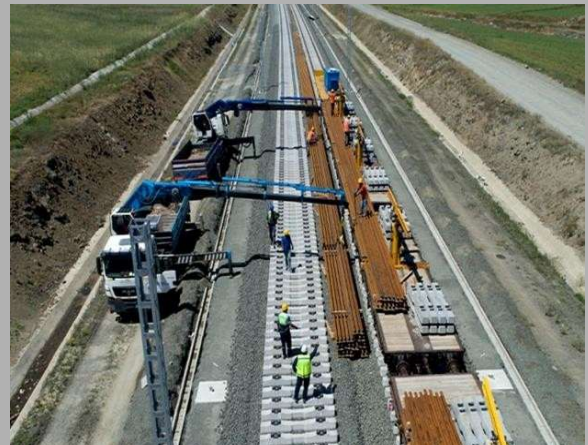
TCDD HIGH SPEED RAILWAY PROJECTS ANKARA/KAYAŞ- YOZGAT/YERKÖY SECTION SUPERSTRUCTURE WORKS
