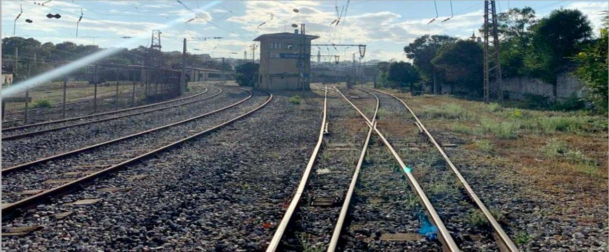
KAZLIÇEŞME-SİRKECİ URBAN TRANSPORTATION AND RECREATION FOCUSED TRANSFORMATION PROJECTS RAILWAY TRACK AND TURNOUT DISASSEMBLY WORKS
