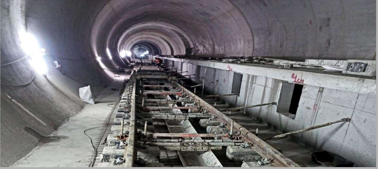
BAŞAKŞEHİR-KAYAŞEHİR METRO LINE CONSTRUCTION AND ELECTROMECHANICAL SYSTEMS SUPPLY, INSTALL AND COMMITIONING WORKS TRACK INSTALLATION CONSTRUCTION WORKS
