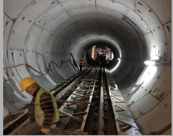
AKM – KIZILAY METRO LINE SUPERSTRUCTURE WORKS (ANKARA)
