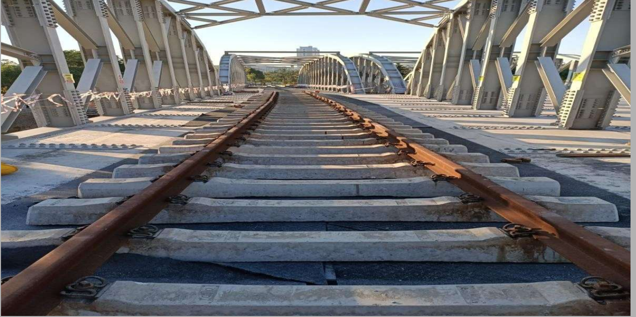
M3 KIRAZLI AKIRKÖY İDO METRO LINE SUPERSTRUCTURE WORKS
