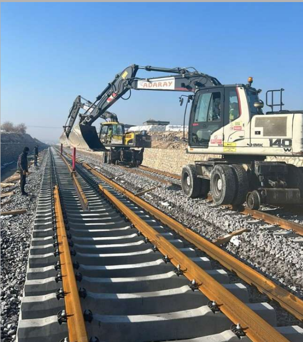
KARAMAN-ULUKİŞLA FAST TRAIN PROJECTS STATION LINES SECURITY TUNNELS AND PROBABLY STRUCTURES CONSTRUCTION WORKS
