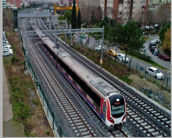
KKC MARMARAY PROJECTS ( İSTANBUL ) GEBZE-HALKALI SUBURBAN LINE CONSTRUCTION AND ELECTROMECHANICAL SYSTEMS EUROPE SECTION SUPERSTRUCTURE WORKS
