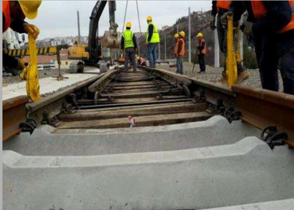
TCDD-GÜLERMAK-KOLİN-KALYON GAZİRAY PROJECTS SUPERSTRUCTURE WORKS (GAZİANTEP)
