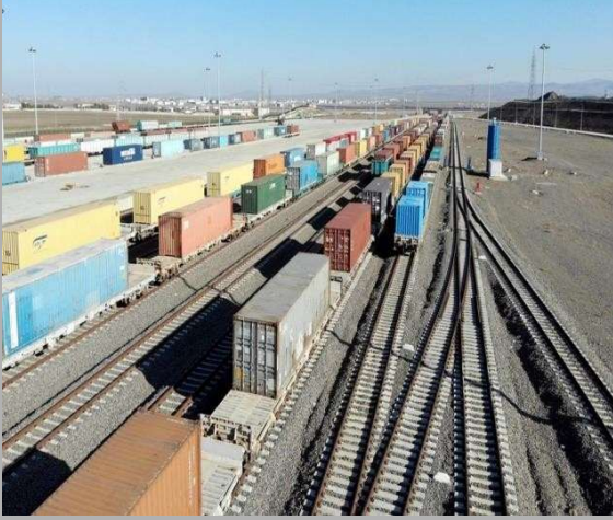
KARS LOGISTIC CENTER AND RAILWAY (DOUBLE GAUGE) CONNECTION WORKS
